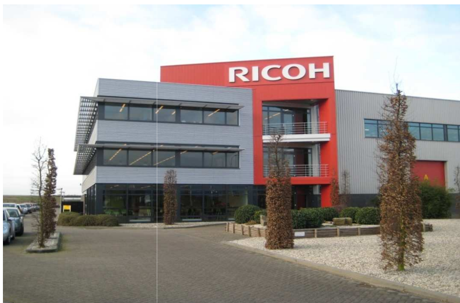
The vast Ricoh distribution centre in Bergen op Zoom (West-Brabant) was part of the Prologis portfolio sold to AEW Europe in the first half of 2009.
